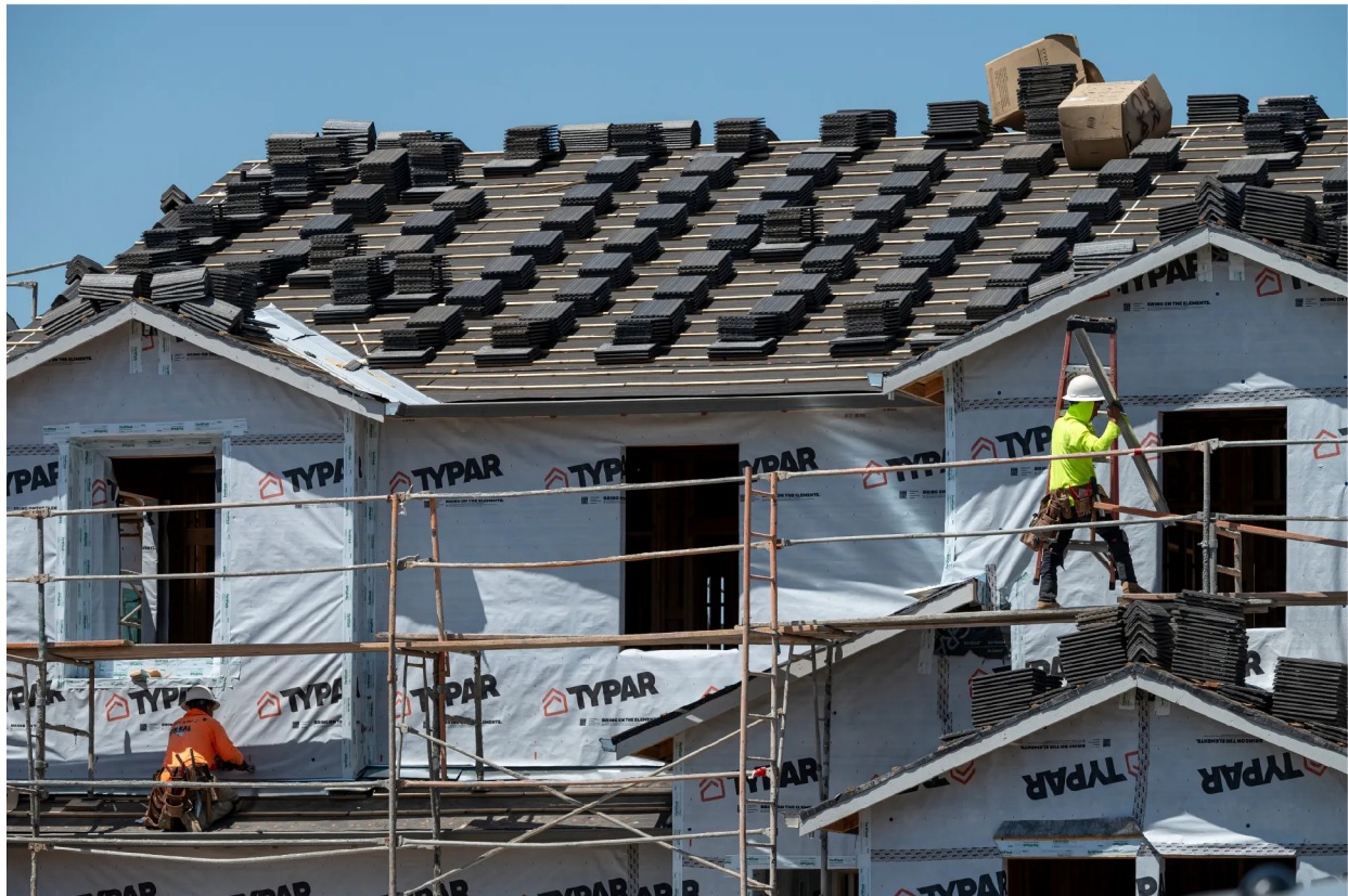
Homes under construction at a housing development in Rancho Cordova, California. Photographer: David Paul Morris/Bloomberg
